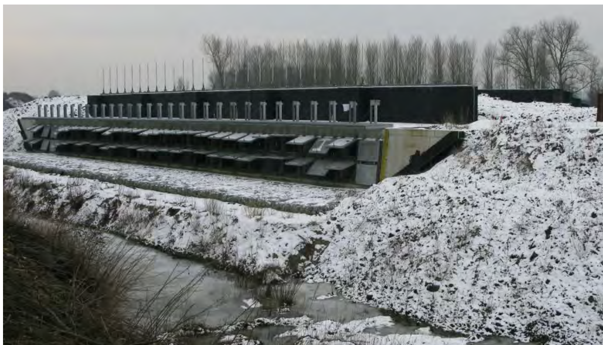
Plate 1: One of the Kruibeke sluices during construction.
